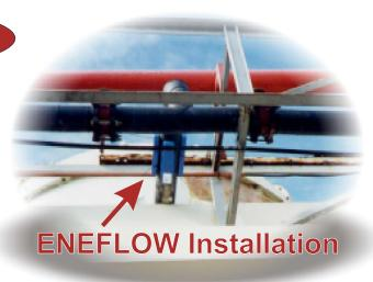
This major starch producer in Thailand had an on-going problem with severe calcium carbonate scale build-up in their cooling tower sprinkler pipe.
